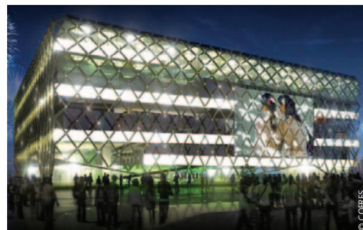
Constructed entirely of recyclable materials, the France Pavilion is a shining example of green design.
